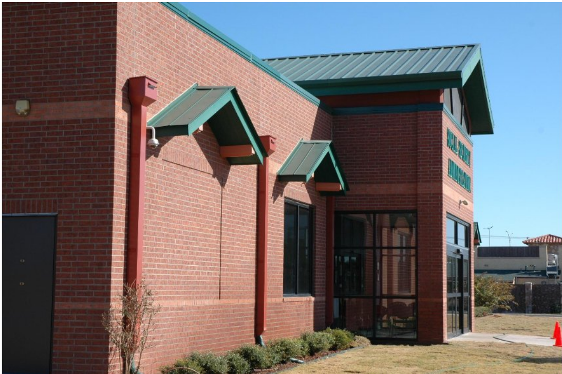
Vies of brick exterior and the standing-seam roof.
