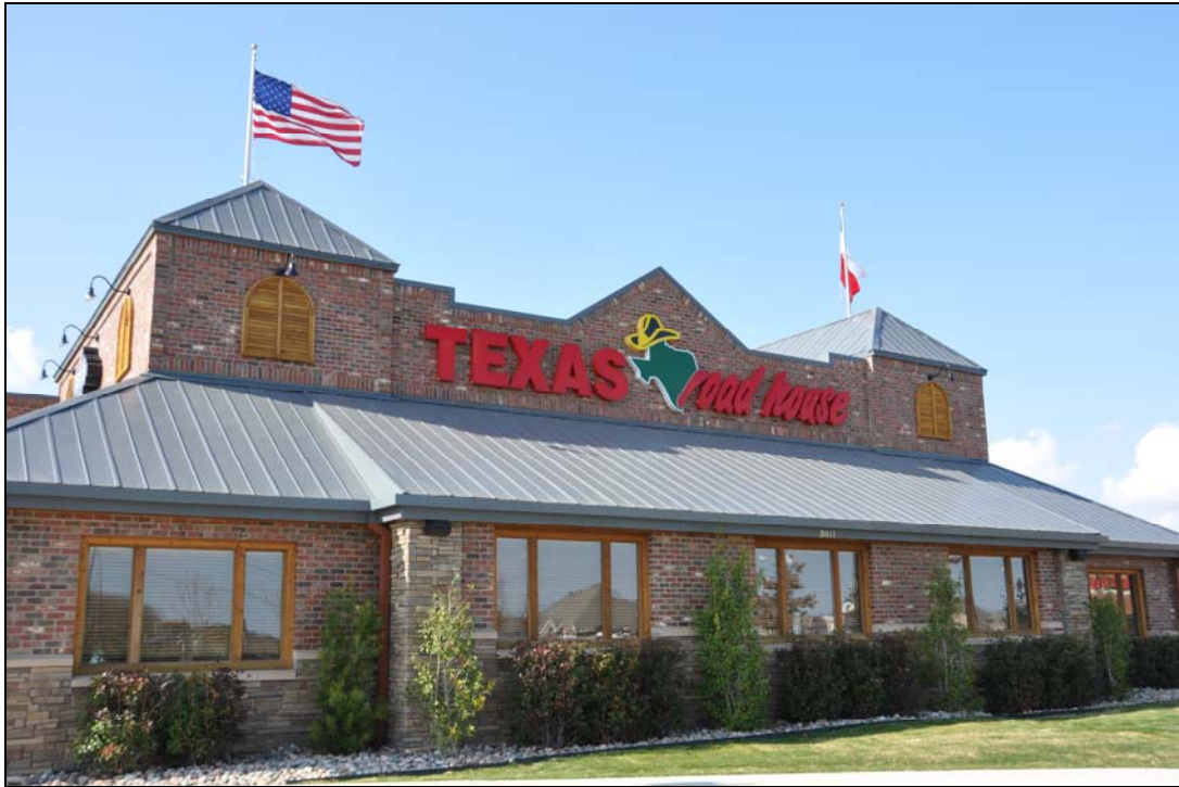
This Texas Road House Restaurant characterizes the upscale retail market.
